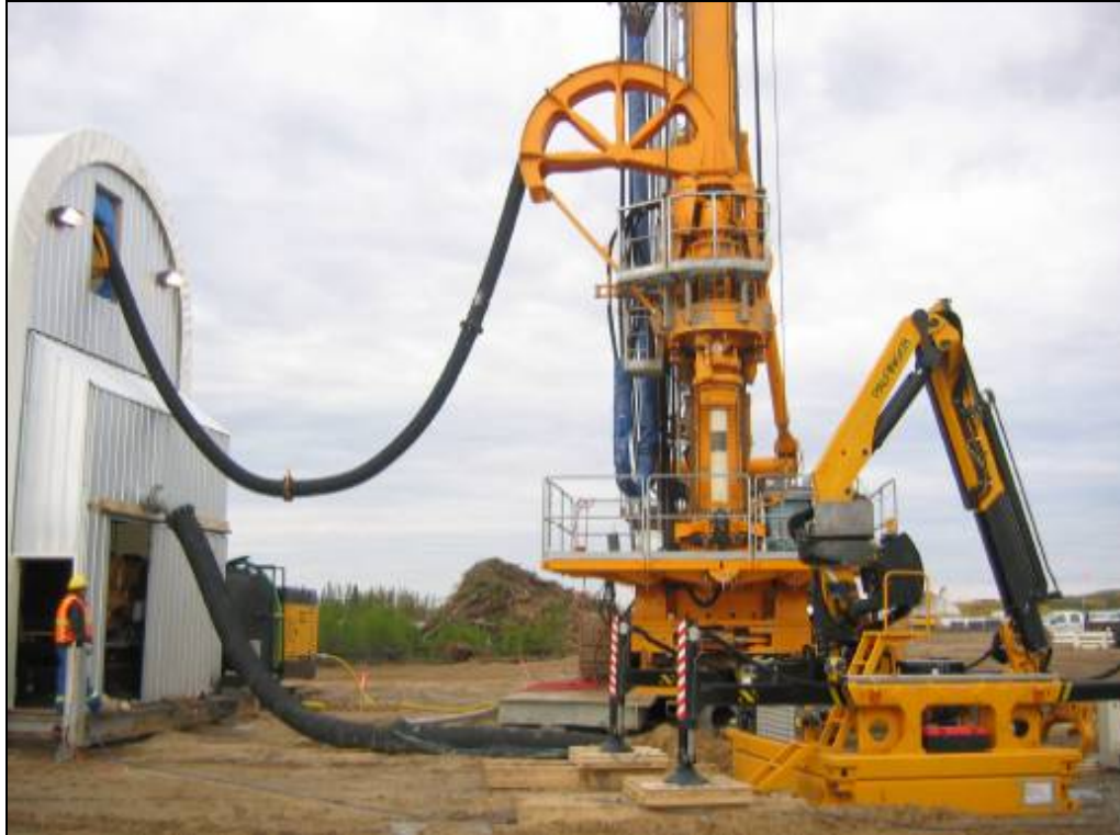
Figure 11-4: Bauer BG-36 Drill Rig
