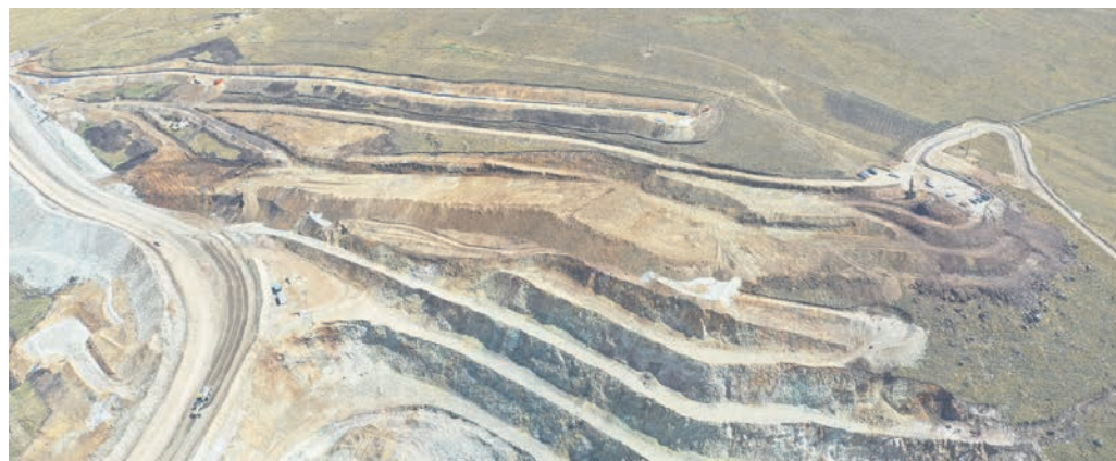
Pampacancha is a high-grade copper and gold satellite deposit located approximately seven kilometres from Hudbay's Constancia mine and processing facilities in Peru. SUPPLIED
